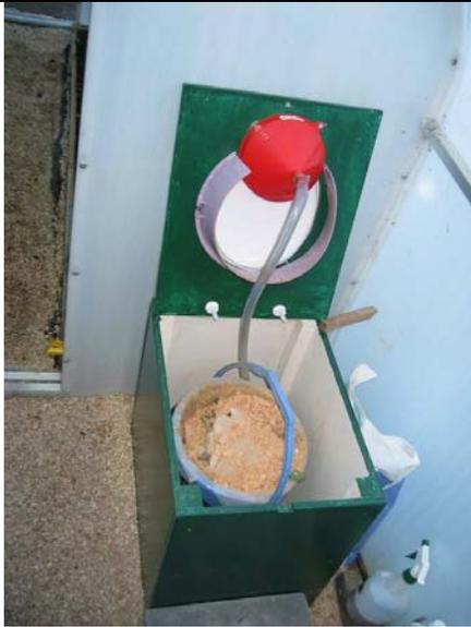
Photo (a) - my simple urine separating pan (using plastic funnel) with lid up
