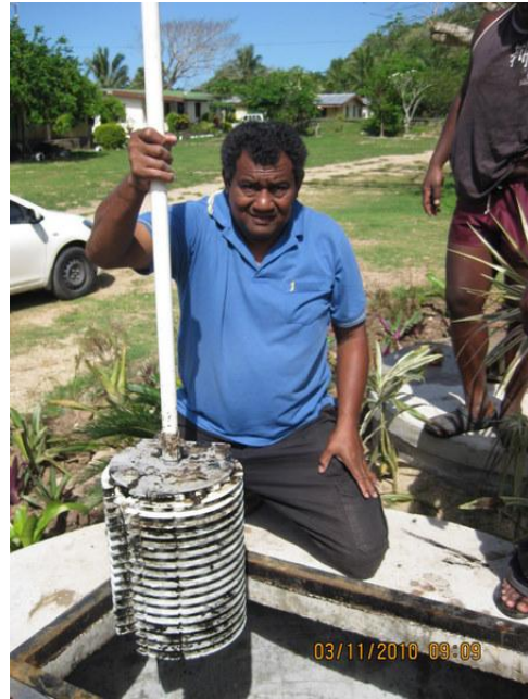
12. Votua Village wastewater pump sump filters being inspected.
